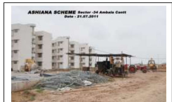
Under construction 1640 dwelling units at Ambala Cantt.
